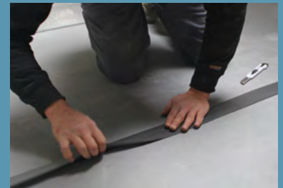
Insure the tightness with the Stickelfoam 25/70
