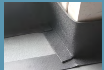
Place the strip L-foam sides against the wall
